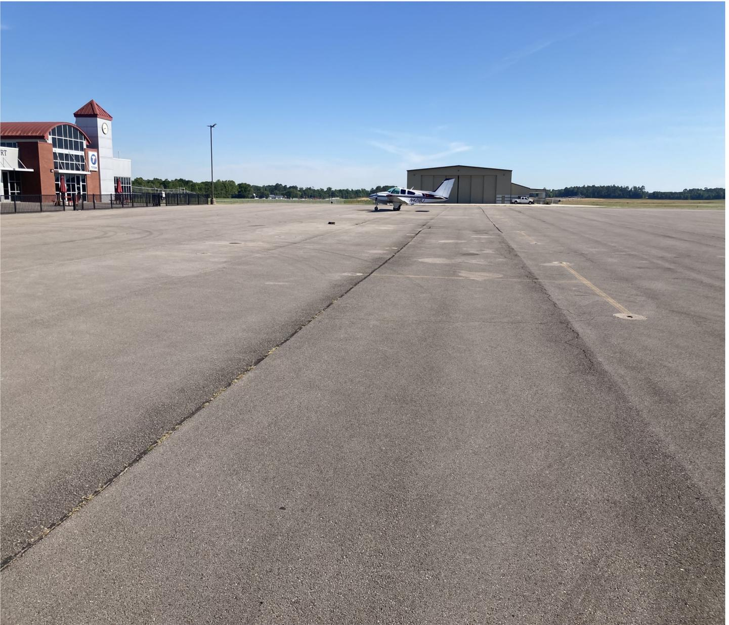
The Terminal Apron is in **FAIR** condition due to minor cracking and vegetation growth.
