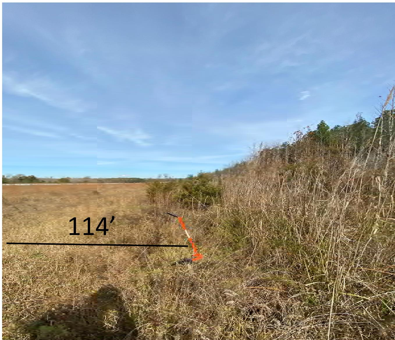
**Violation:** Primary Surface **DOES NOT MEET** state licensing standards. Ensure grass and trees are cut and removed from of the Primary Surface. 114' to runway centerline; 125' from centerline is required.
