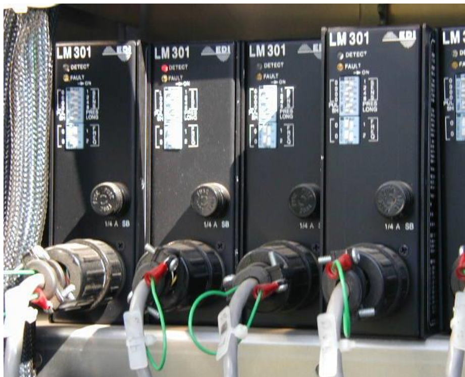
Figure 12.6 – Single channel vehicle loop detectors
