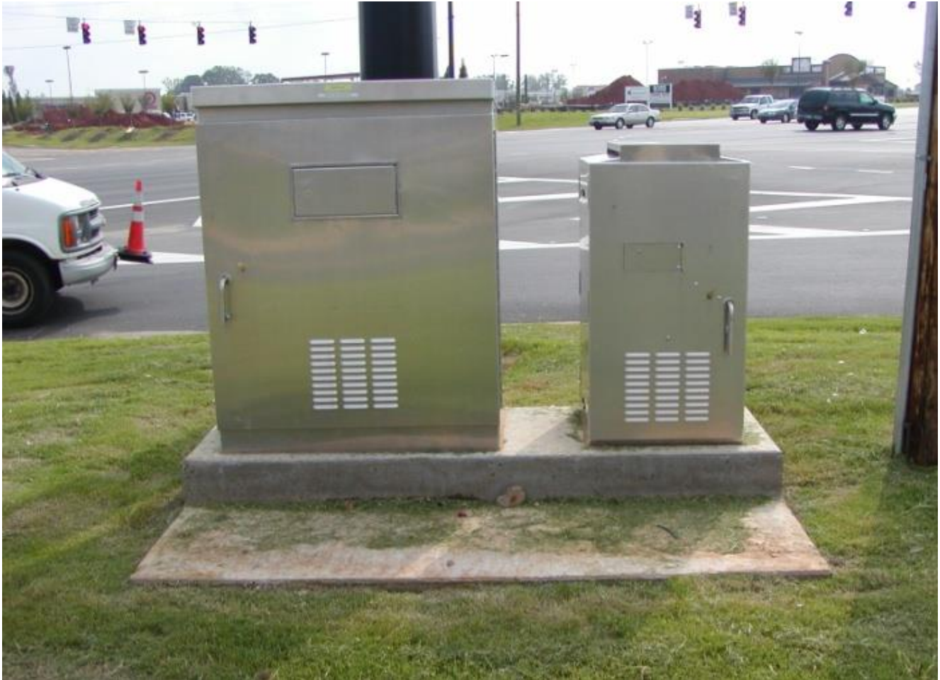
Figure 12.11 – Typical installation of UPS in separate cabinet
