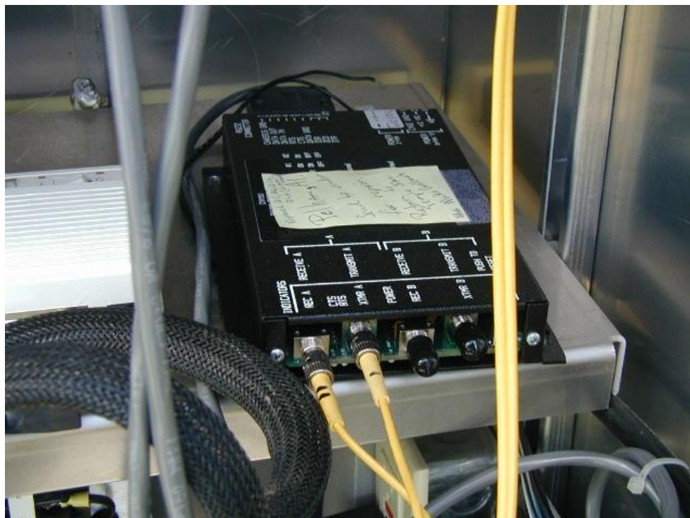
Figure 12.8 – Fiber optic modem (external)
