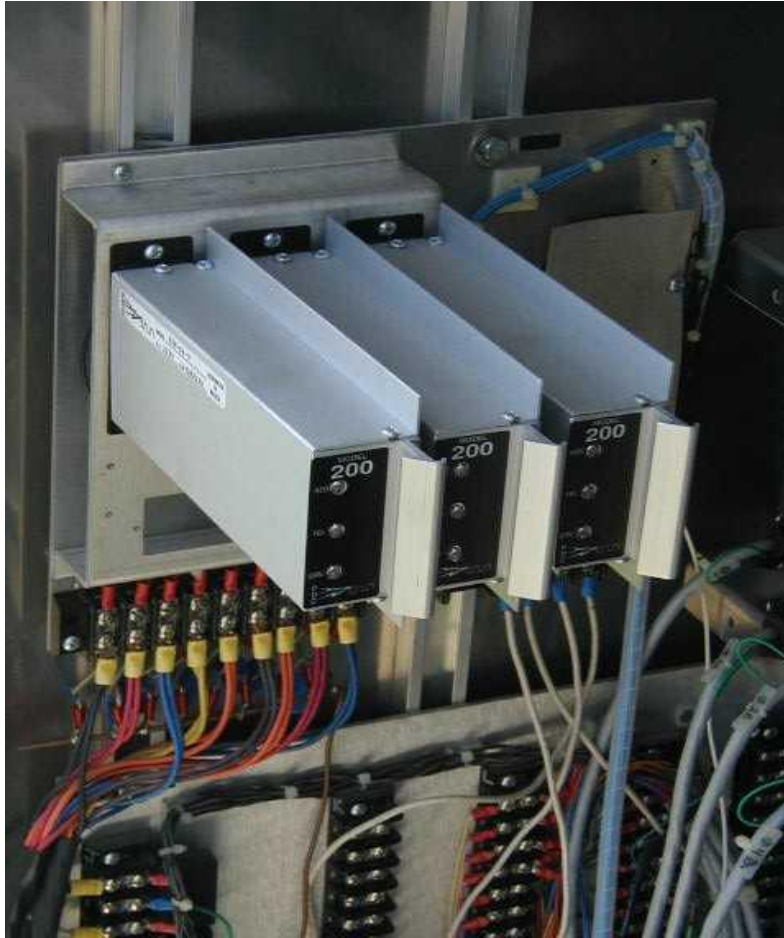
Figure 10.1 – Typical hardwire interconnect panel
